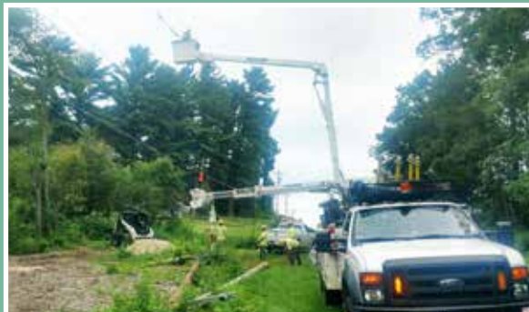
Overhead three-phase was rebuilt in Tunnel City.
