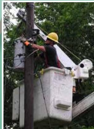
Erick Flock received his Journeyman Lineman Certification.
