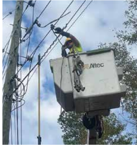
Dalton placing protective grounds to allow for safe working conditions.
